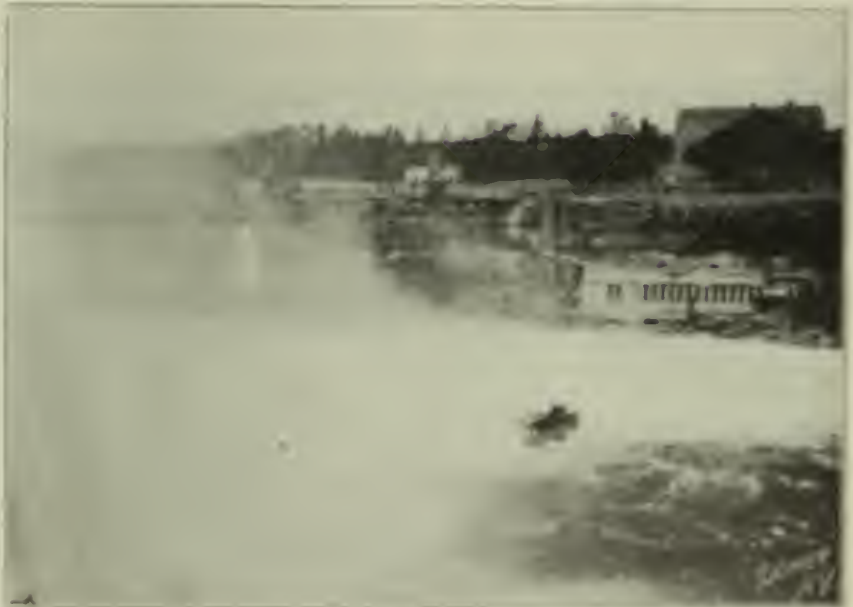
FIG. 4. WITH THE SURFACE BELOW COMPANY'S POWER HOUSE COVERED WITH ICE.
